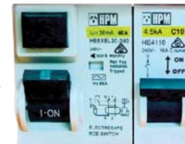
**Figure 6.23:** A miniature circuit breaker (MCD) and residual current device (RCD) are indispensable when water and electricity are in close proximity.
